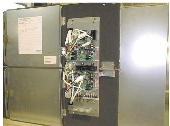
②Remove all harnesses connected to the circuit board.
