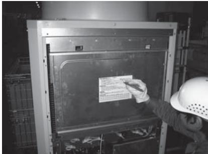
⑩ Closing the valve on the connecting port to the refrigerant circuit
